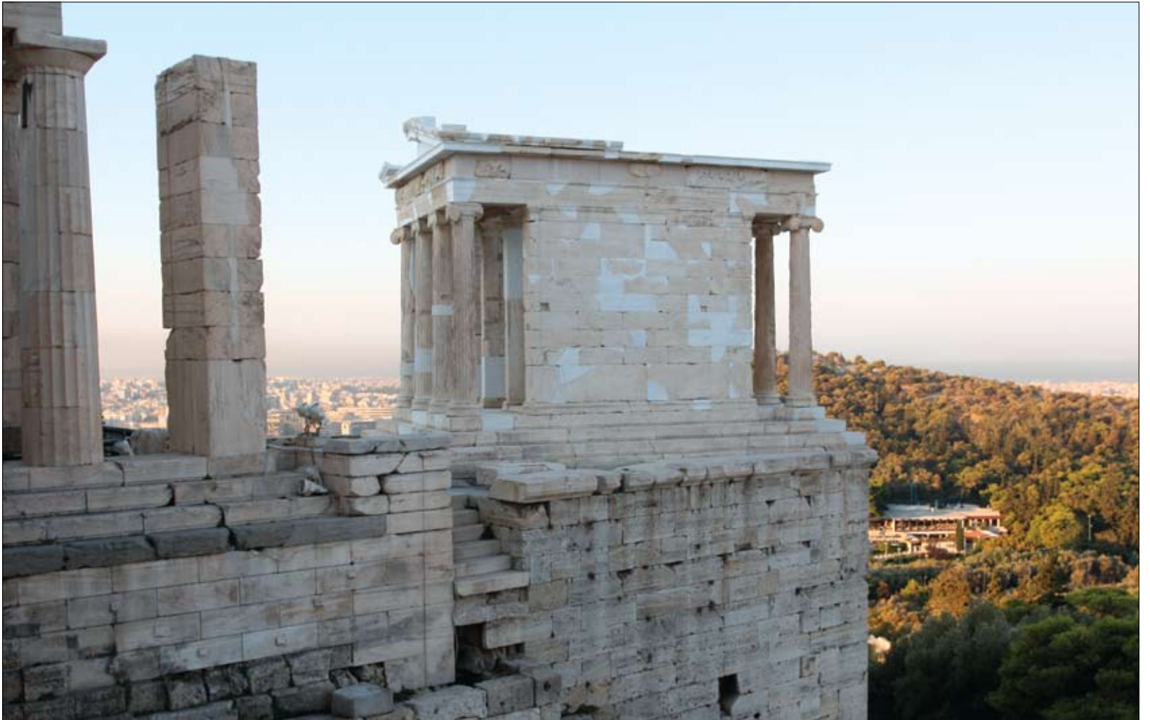
60. The temple of Athena Nike after its restoration. View from the northeast.
