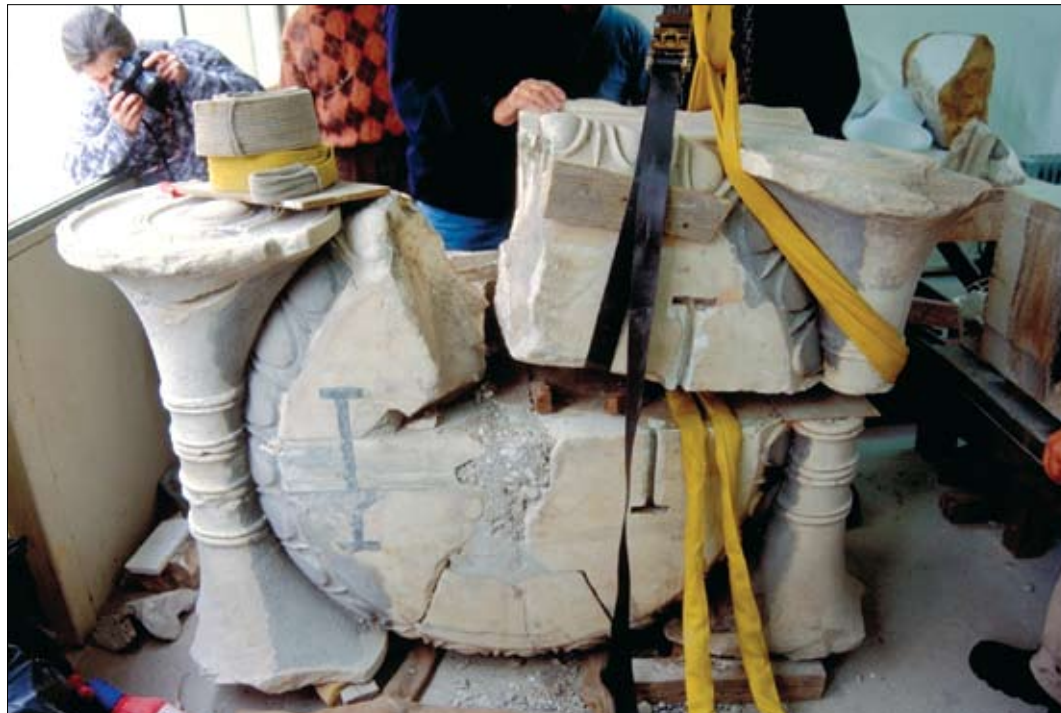
50. Dismantling the column capital of the Balanos anastelosis in the Propylaea laboratory.
