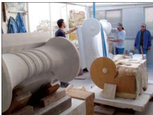
51. Carving the Ionic capitals from new marble in the Propylaea laboratory.
