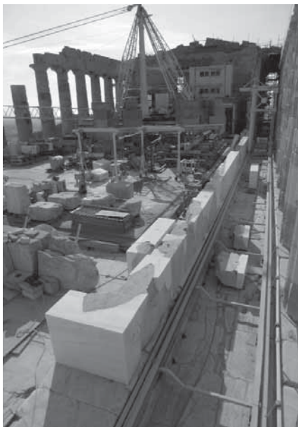
Restoration works of the north wall first course of the Parthenon cella. Photo R. Christodouloupoulou, 2016
