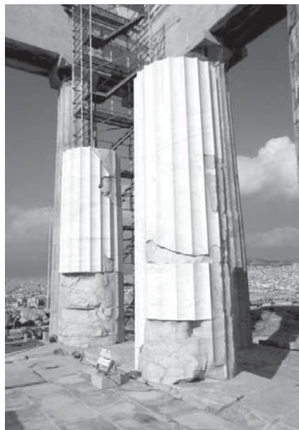
The two columns of the Parthenon pronaos after the completion of carving the drum flutes. Photo R. Christodouloupoulou, 2016
