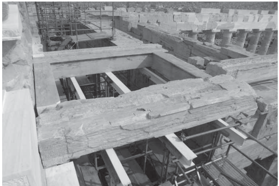
View of the two repositioned beams from the ceiling of the Parthenon west colonnade. Photo P. Christodouloupoulou, 2016
