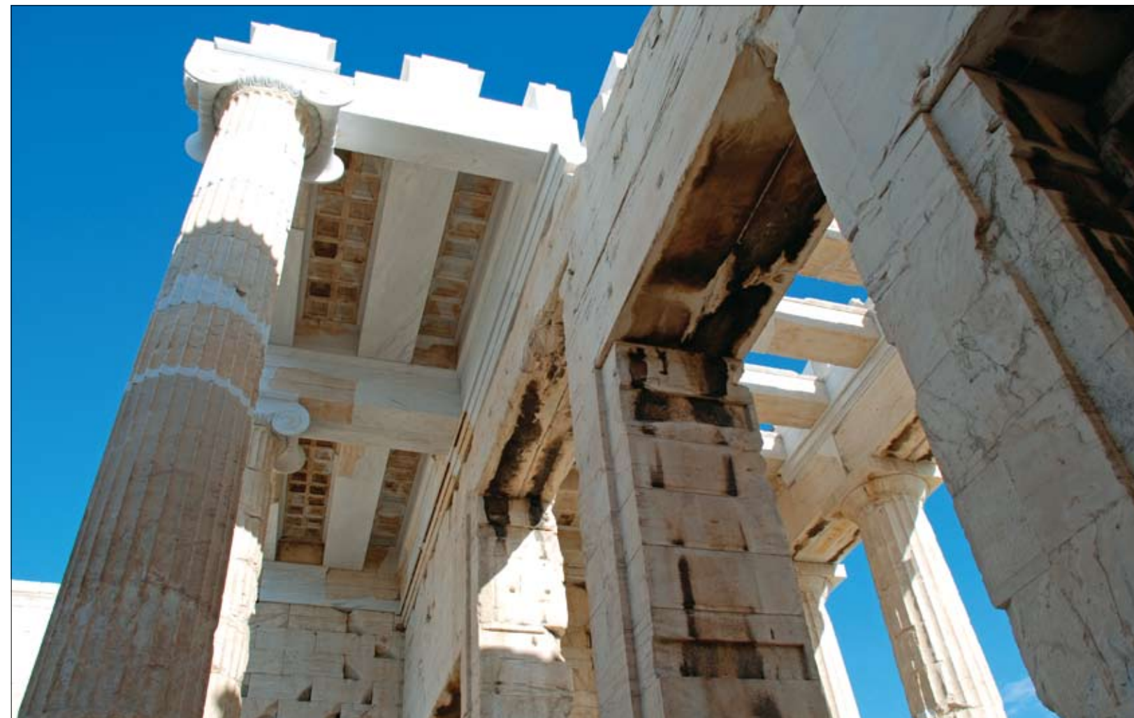
57. Propylaia. The restored ceilings of the west hall and the east portico from the south.
