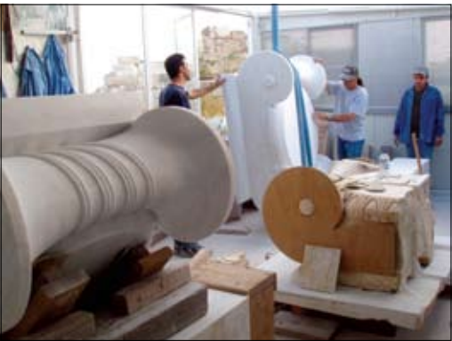
51. Carving the Ionic capitals from new marble in the Propylaia laboratory.
