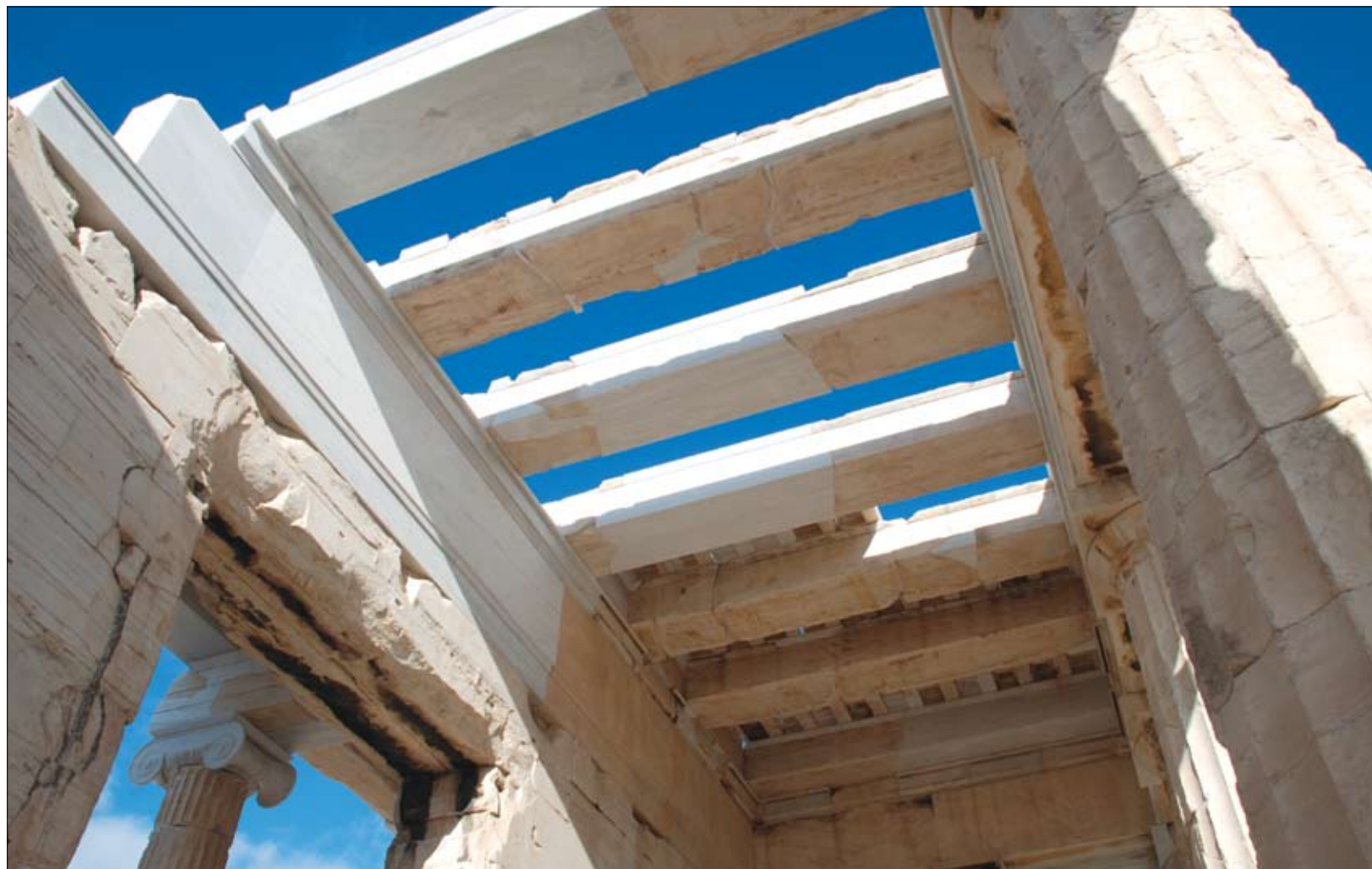
58. Propylaea. The ceiling of the east portico after anastelosis. View from the south.
