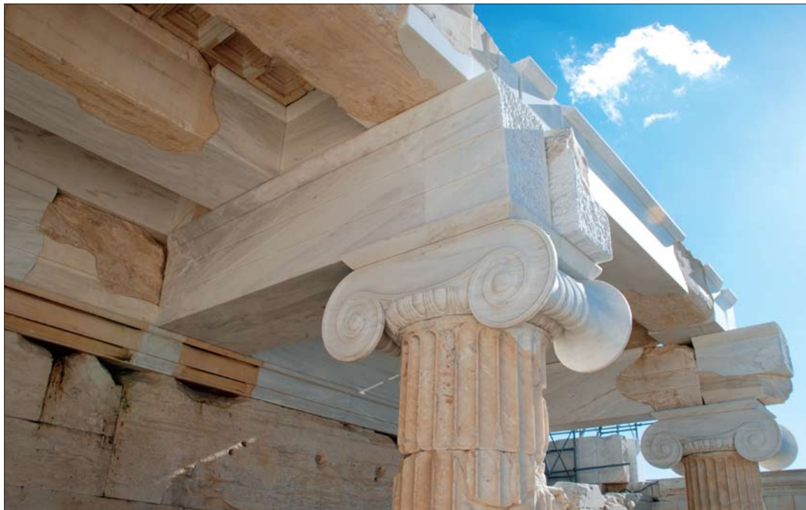
56. Propylaia. The ceiling of the west hall after anastelosis. Visible are the two copies of the Ionic column capitals. View from the northwest.
