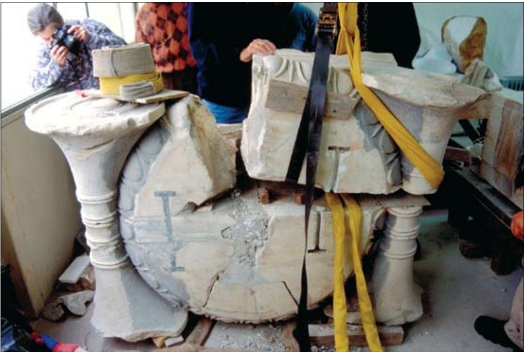
50. Dismantling the column capital of the Balanos anastelosis in the Propylaia laboratory.
