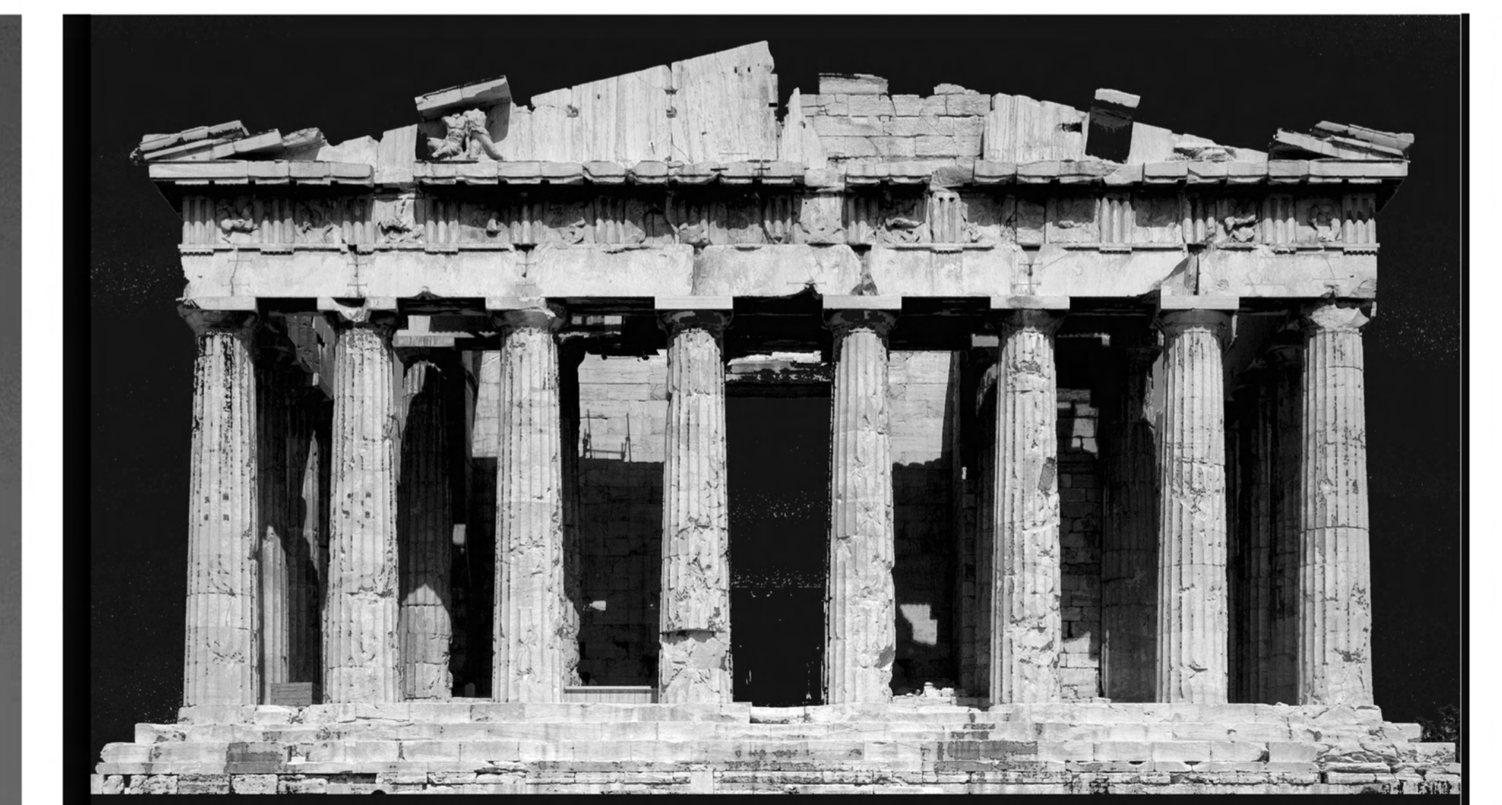
The west side before the beginning of the current restoration programme – Photo S. Mavrommatis
